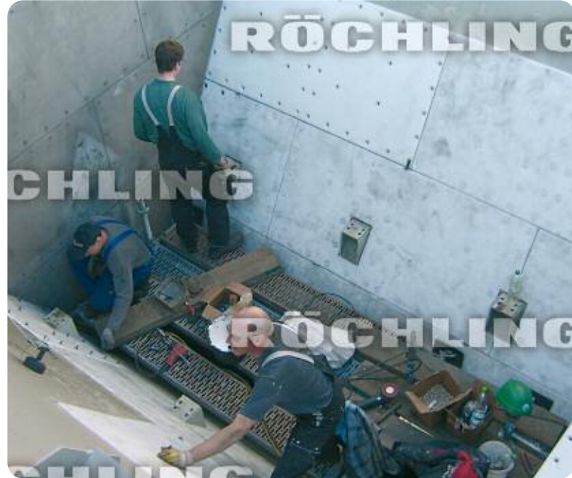
Stud-welding process: lining a hopper
